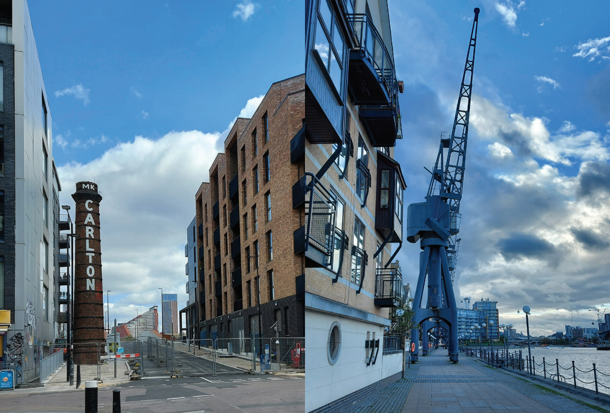
Fig. 6: Retained chimney in HWFI (April 2021).
